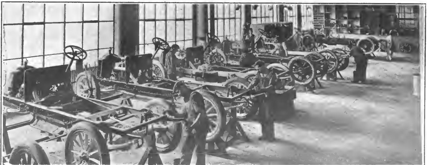
Fig. 5—Chassis painting section. Each group of painters devotes its time to work on one particular part of the Packard machine
